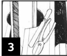
3 Cut out marked portions of roof, filing away sharp edges and install pipe securely in place. Where required, support cut sections of sheet with additional framing to support base.
